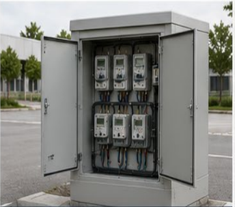
OUTDOOR METER PANEL
