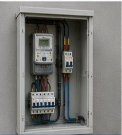
SINGLE PHASE METER PANEL
