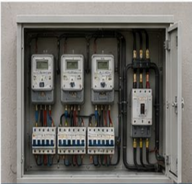
METERING WITH MAIN BREAKER
