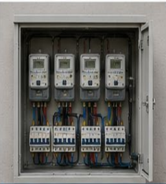
THREE PHASE METER PANEL
