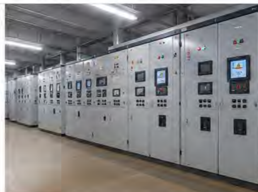
AUTOMATIC POWER FACTOR CORRECTION PANELS Optimize energy efficiency and reduce power losses.
