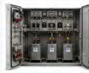
AUTOMATIC POWER FACTOR CORRECTION PANELS Optimize energy efficiency and reduce power losses.
